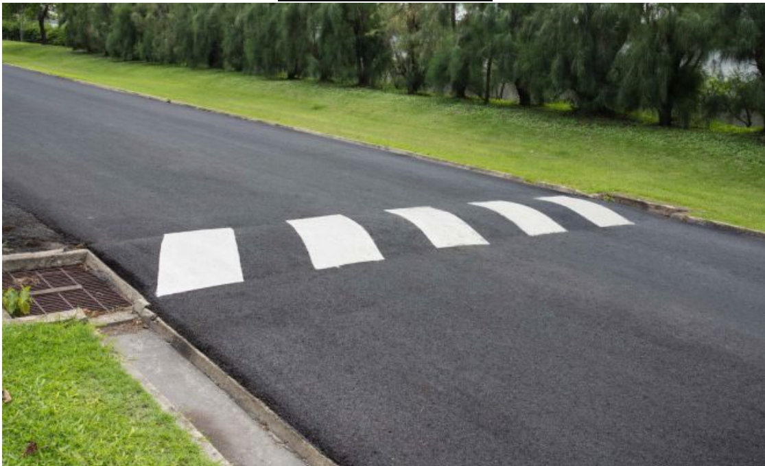
Example of speed hump
